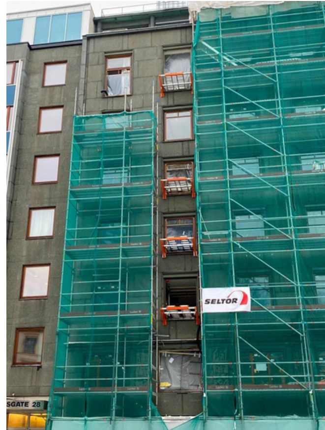
Seltor AS – Office Building KA 23
